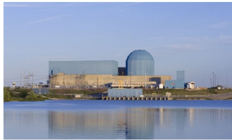
Clinton nuclear plant
