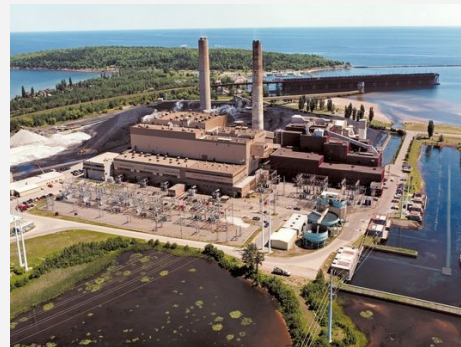
Presque Isle power plant
